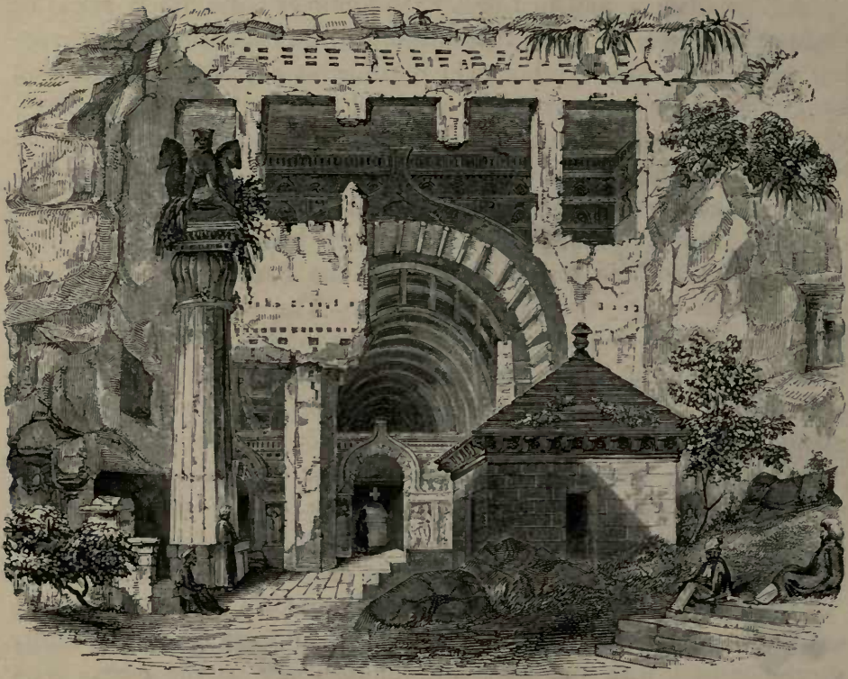
No. 47. Facade of Chaitya Cave at Karle, from a sketch by J. F.
